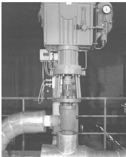
Leak-off valve ZK 213 with compact electro-hydraulic actuator
