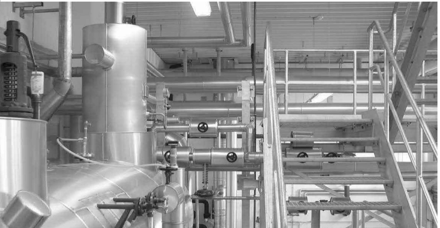
The make-up water and return condensate enter the NDR deaerator dome, which is fitted with a series of welded tray compartments for maximum trickling. Heating steam is fed from below into the NDR deaerator dome, which is mounted on top of the SW feedwater tank. The deaerated make-up water and return condensate flow directly from the deaerated dome into the feedwater tank. A steam injector installed in the lower part of the feedwater tank is used to heat up the feedwater to approx. 107 °C.
