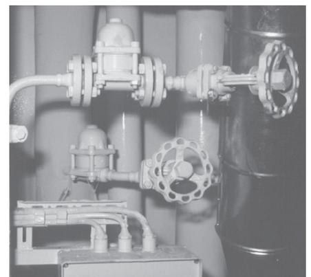
*Tank-heating system equipped with BW on an ore carrier*
