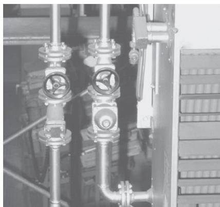
*BW installed downstream of an air heater (space heating)*
